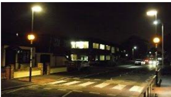
Combined Belisha beacon & streetlamp illuminating a zebra crossing at night. (Photo credit: The Ranty Highwayman/@RantyHighwayman)
