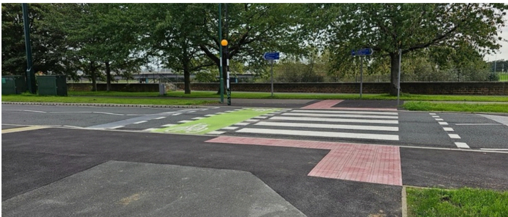
A parallel crossing in Nottingham. The coloured cycle part of the crossing highlights to drivers that this is different from a plain zebra crossing. (Photo credit: Kevin S/@kevjs1982)
