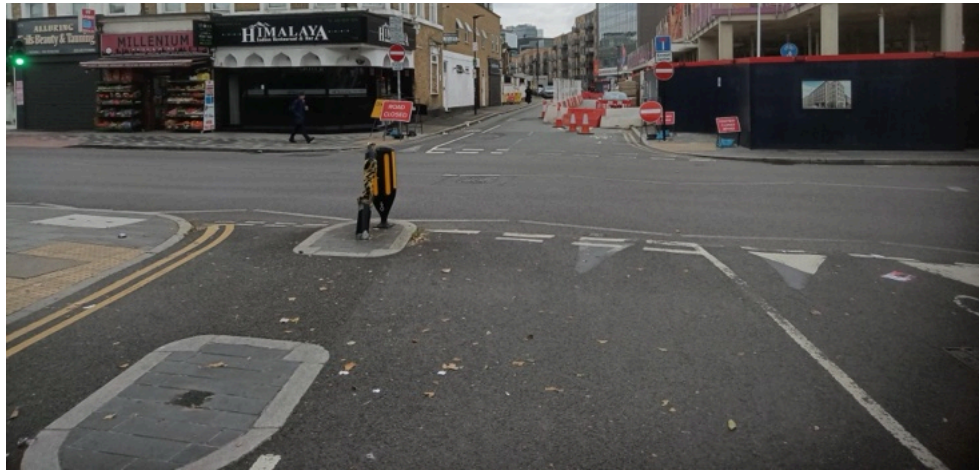
Looking west from Manbey Grove towards Grove Crescent Road. Note the redundant island to protect the (now-unnecessary) contraflow. Photo credit: Nigel King
